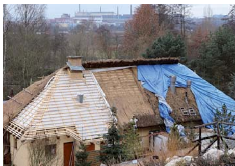
Oprava střechy restaurace Kiboko Repairing of the roof of our Kiboko restaurant
